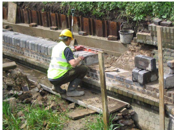
The towpath wall is being built along the canal at Newhouse.
