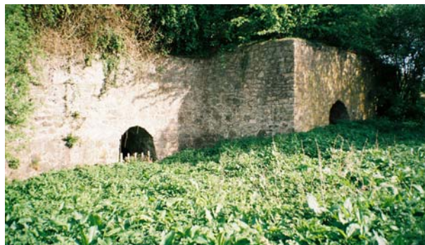
Limekilns at Belan
